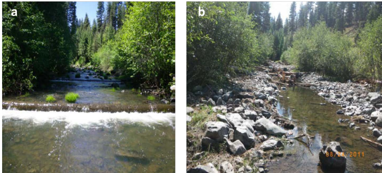
Figure 1. (a) Example of Camp Creek reach with log weir installation. Photo taken 6/20/2010 (b) Reach after log weir removal. Photo taken 8/24/2011.
