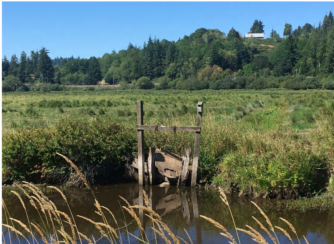
Figure 2. An older style of tide gate found in Oregon. (Photo by Coquille Watershed Association.)
