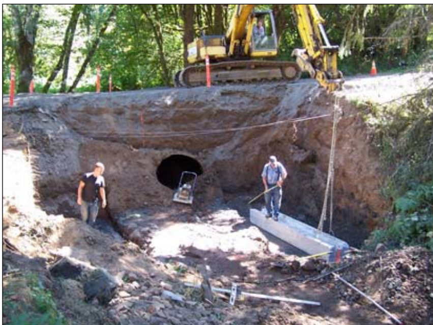
Figure 5a. Opportunistic photo documenting the installation of a culvert.
