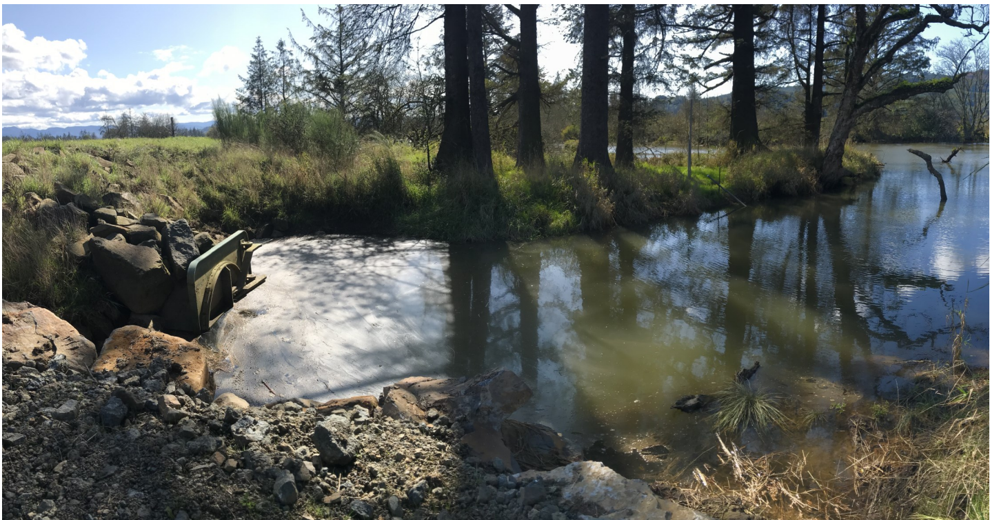
A side-hinged tide gate near the Southern Flow Corridor project reconnects a channel to the Tillamook River. The tide gate is installed in a setback-levee to protect the pasture from high tides, while allowing it to drain at low tides. Source: OWEB
