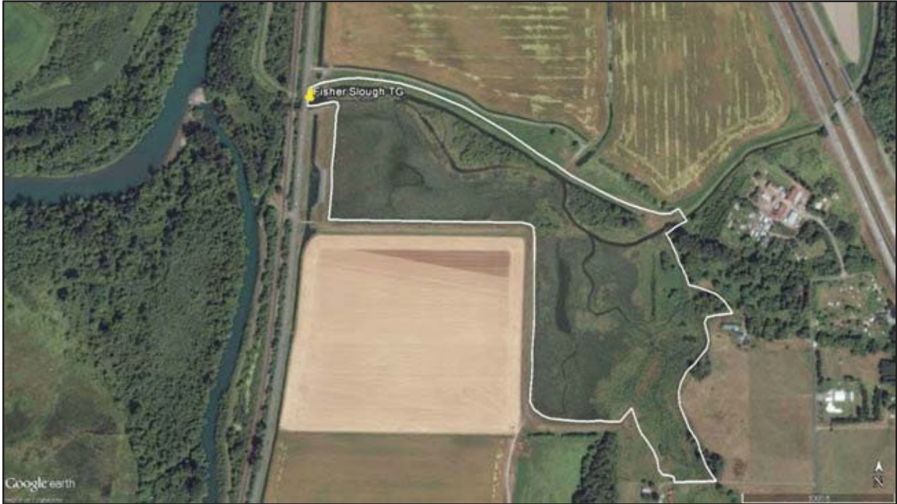
Aerial Images: Fisher Slough after project (8/3/2016).
