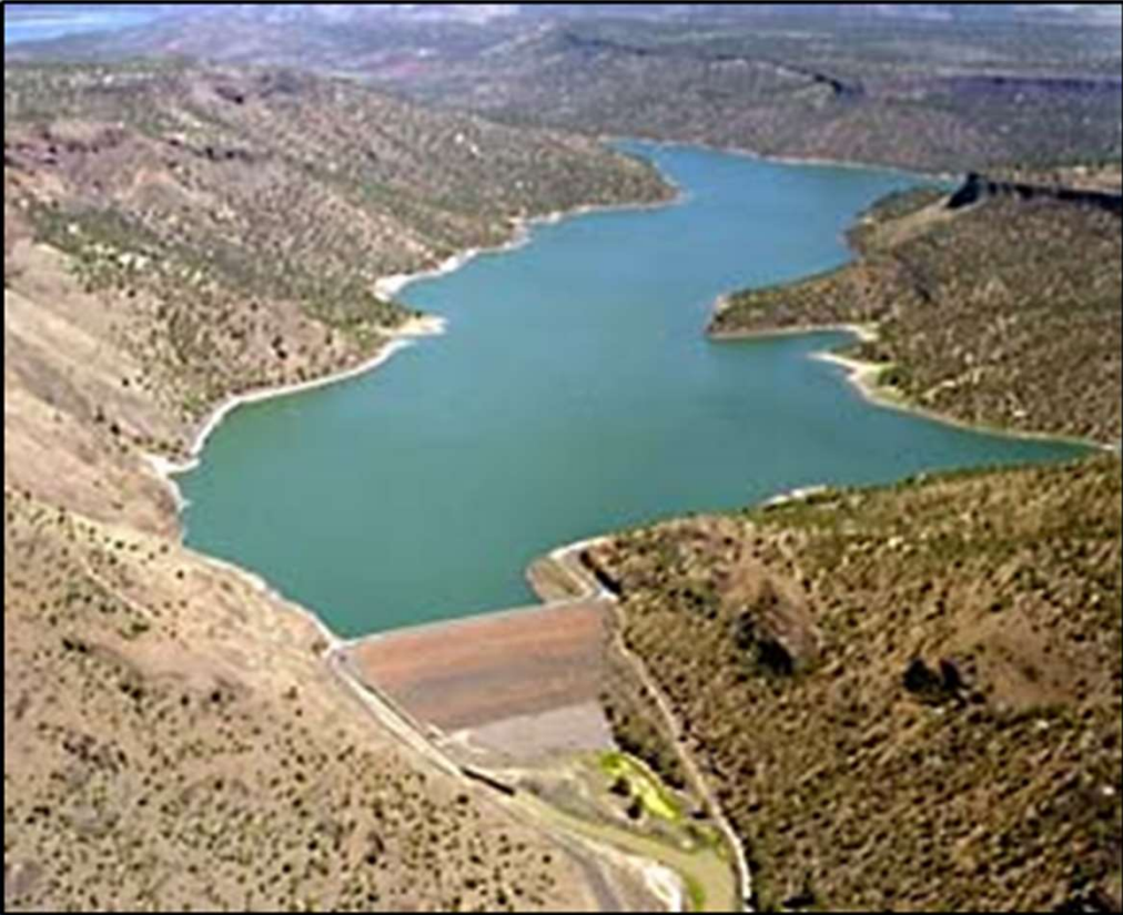
Reservoir storage (full amount)
