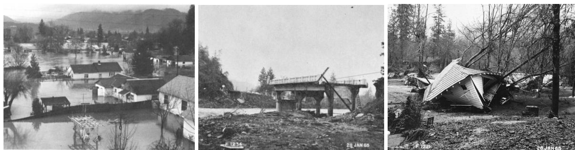
Figure 15. Photos of Rogue River flooding and damage, December 1964.
