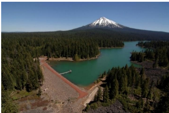
Figure 18. Photo of Fish Lake Dam, looking toward Mount McLoughlin. Photo: USBR .
