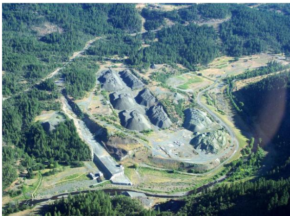
Figure 25. Aerial photo of Elk Creek dam after notching of the dam. Photo: USACE (2022).
