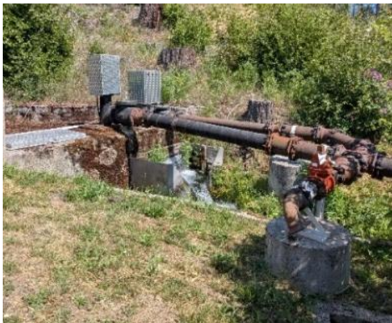
Figure 24. Photo of collection and overflow system at one of the Big Butte Springs. The box captures water springing from the hillside, which then enters a pipe or the overflow.
