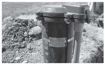
A metal well label, displaying the well ID number, should be on every well.
