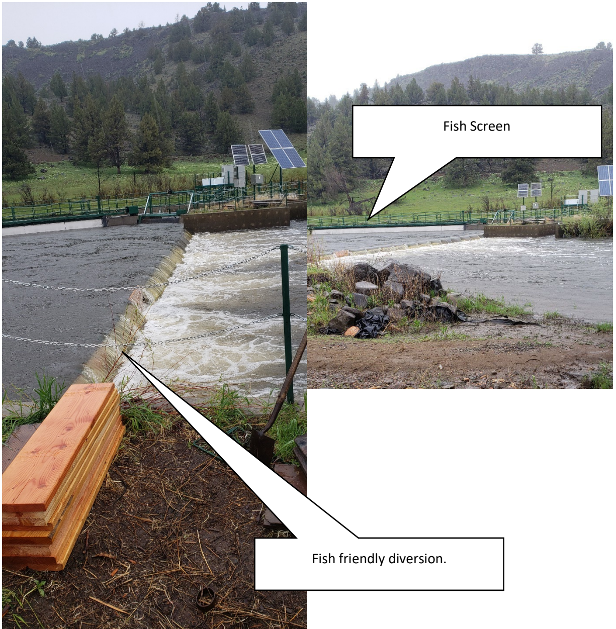
Figure 3. Diversion structure and fish screen where water is diverted from the river into the ditch.
