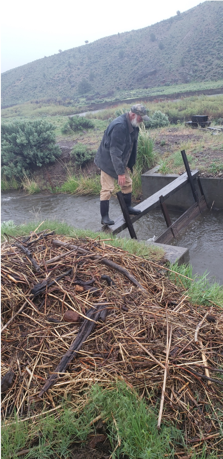
Figure 5. One of the turnouts on the Drewsey Ditch that supplies water to fields below.
