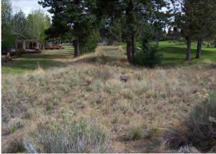
Figure 6-1. A section of nearby Tumalo Irrigation District’s Bend Feed Canal after a piping project.
