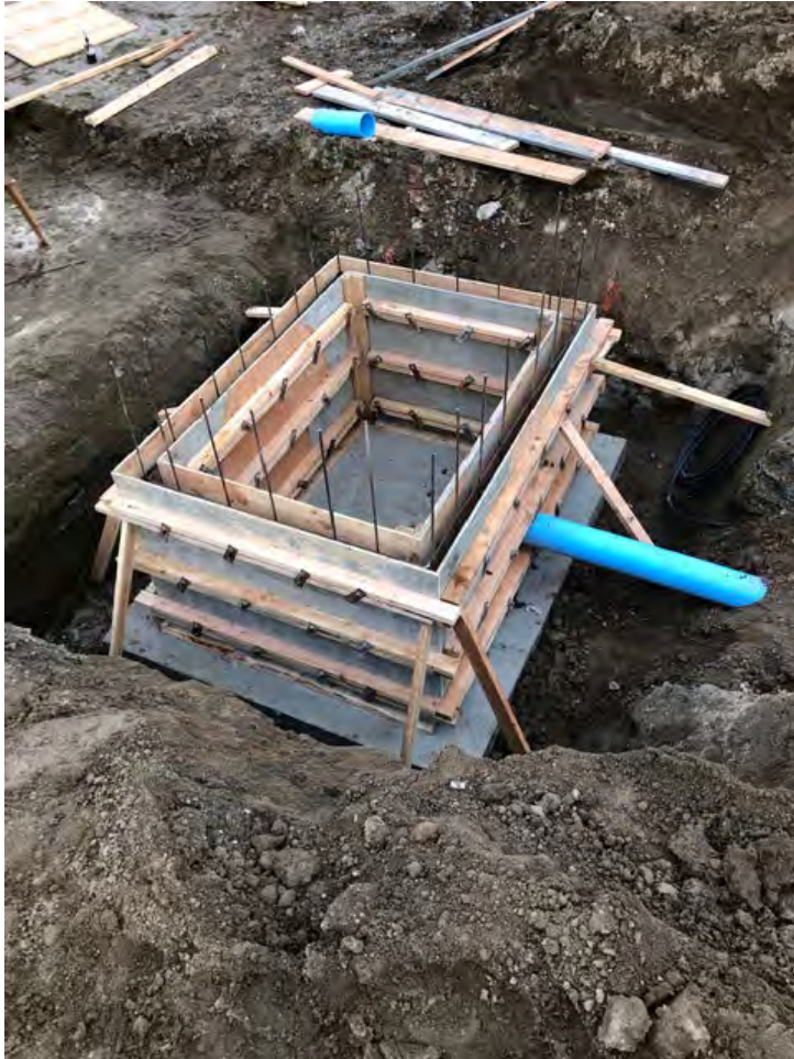
Lateral 273 headgate under construction
