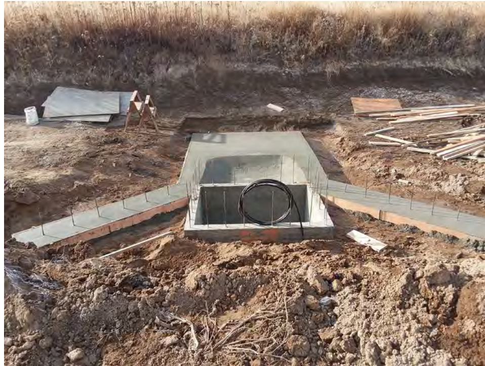
Lateral 273 headgate completed
