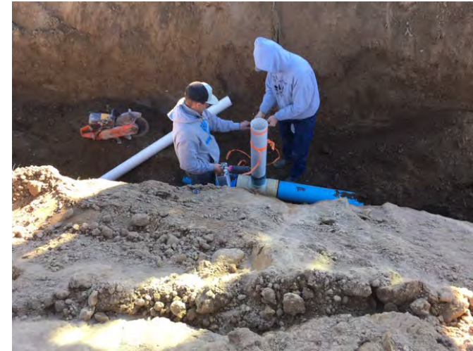
Lateral 273 flowmeter being installed
