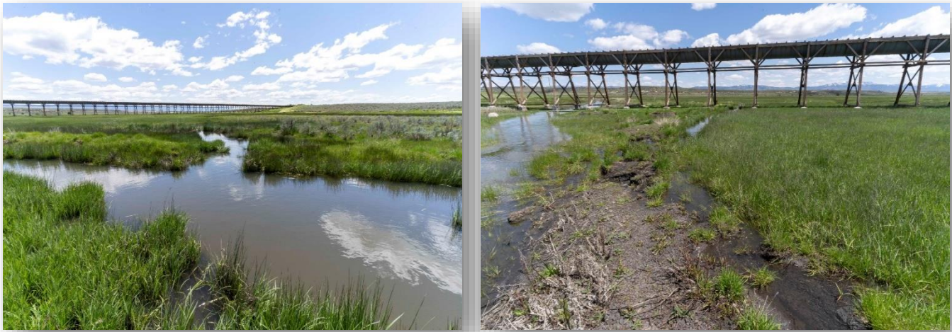
Figure 7. The location of the Site 4 headgate (white arrow) at the upstream end of the earthen berm (left), and the location of the proposed slidegate return pipe (white arrow) at the downstream end of the Site 5 excavated channel segment (right).
