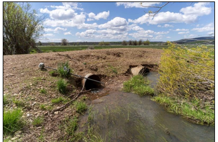
Figure 5. An upstream view of overland flow to the river-left side of the earthen berm (left), and the existing crossing that will be replaced with an armored crossing (right).
