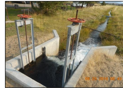
C-9 Sub Lateral Weir, high approach velocity, turbulent, non-uniform velocity at weir crest
