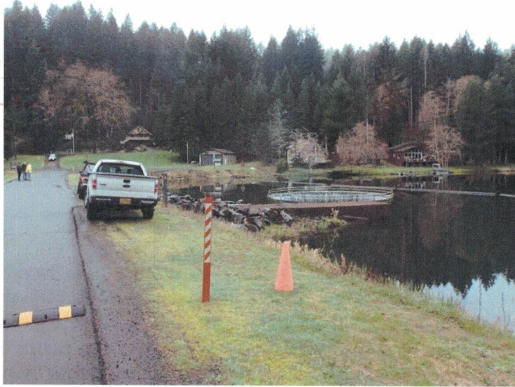
Interior overflow spillway – only spillway
