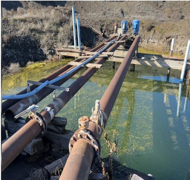
Photo shows dug well with open cover and opening greater than 10 ft. Water in the well is exposed and is a safety hazard.
