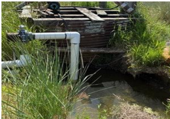
Photo of the casing and seal exposed.
