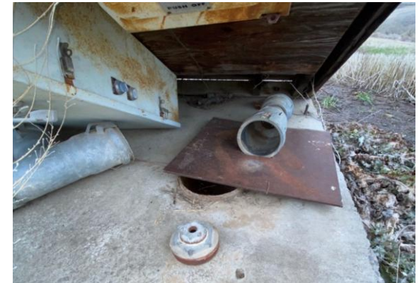
Photo of collapsed well house and open well cover, represents a safety and health hazard.
