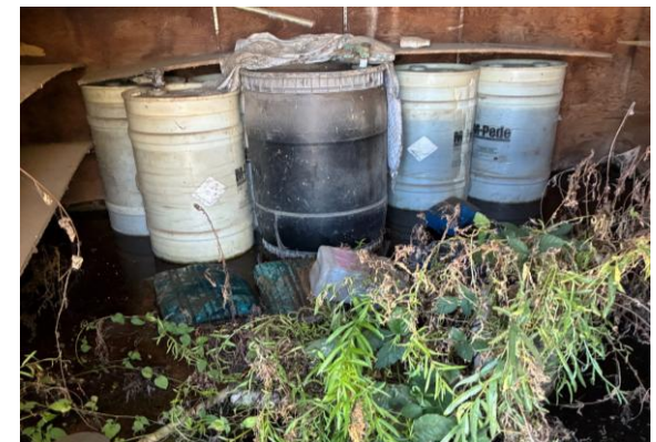
Photo of well house with plants growing inside the building, standing water on the ground, and chemicals being stored.
