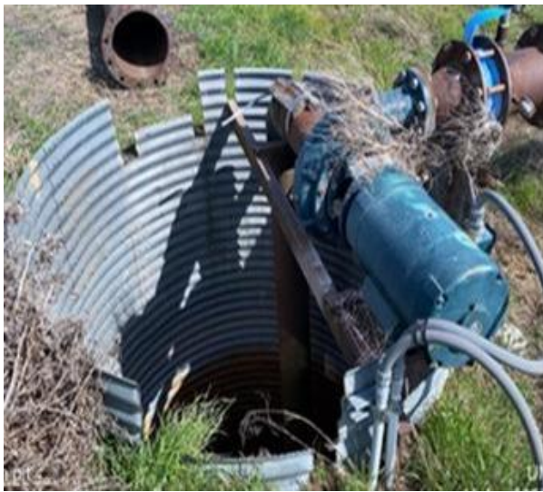
Photo of irrigation pump over an exposed well. Chemicals or animals could enter the well.
