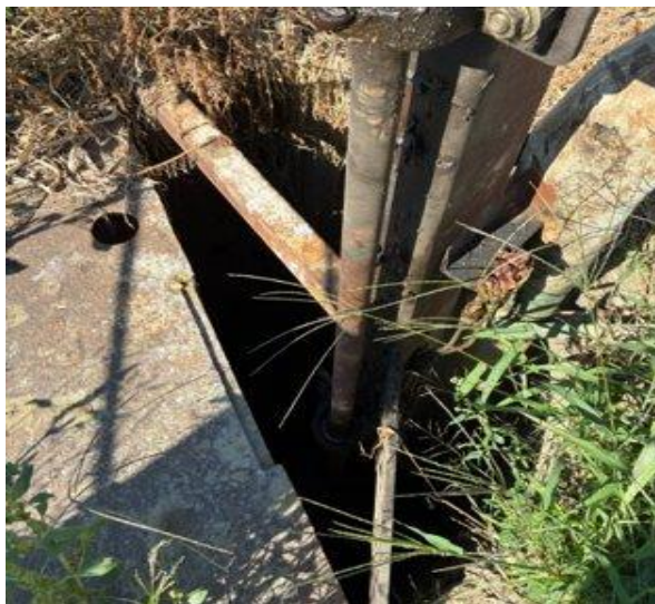
Photo shows partially uncovered dug well.
