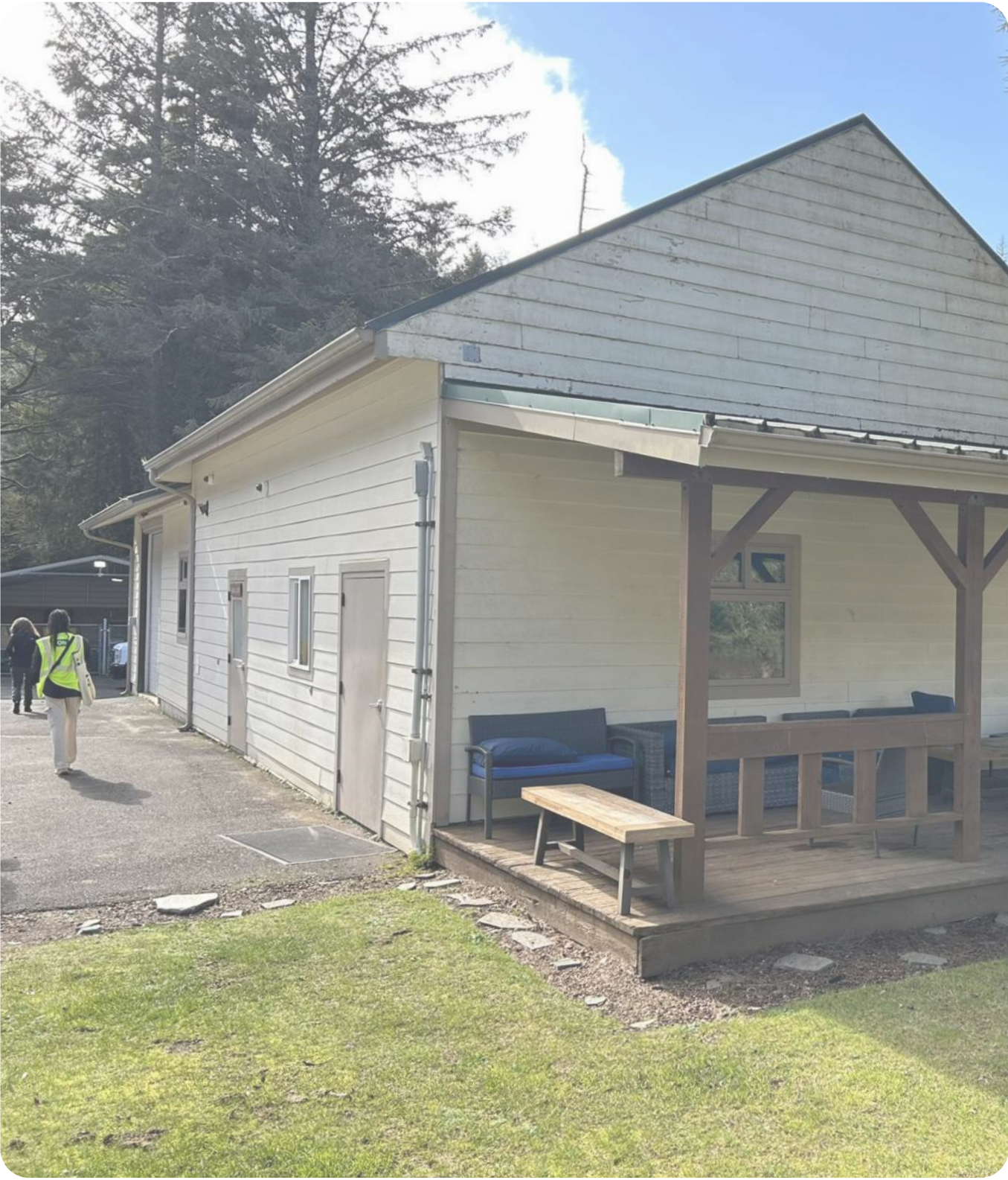
EXTERIOR OF THE SHOP/EXERCISE BUILDING
