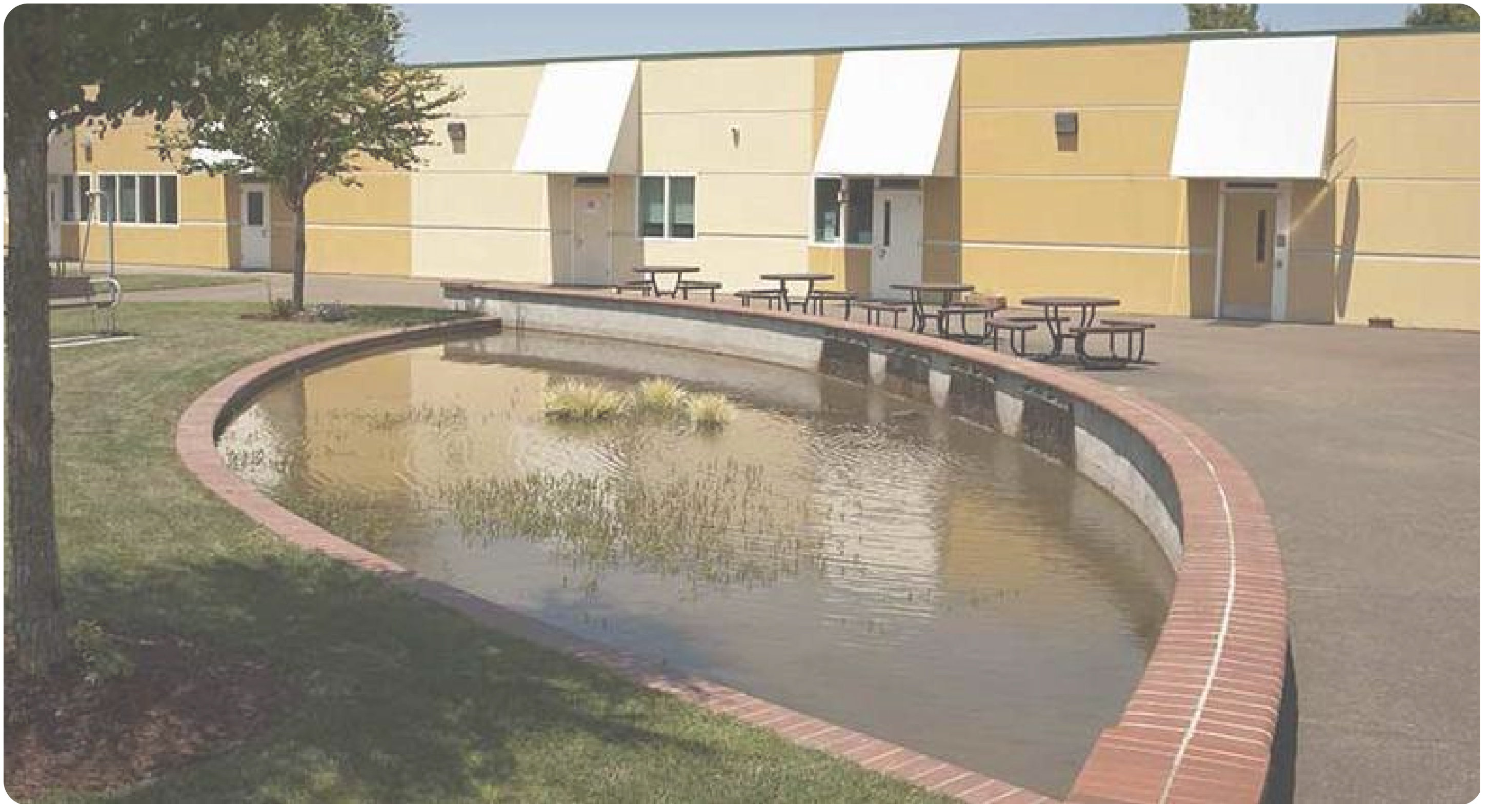
EXISTING VIEW FROM THE INTERIOR COURTYARD AT OAK CREEK YCF
