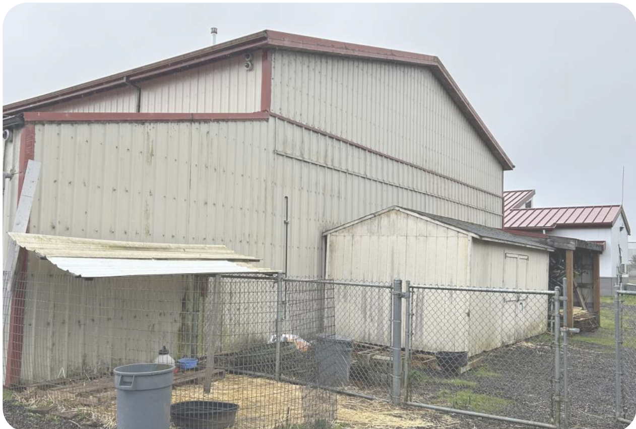
EXTERIOR OF THE RECREATION BUILDING
