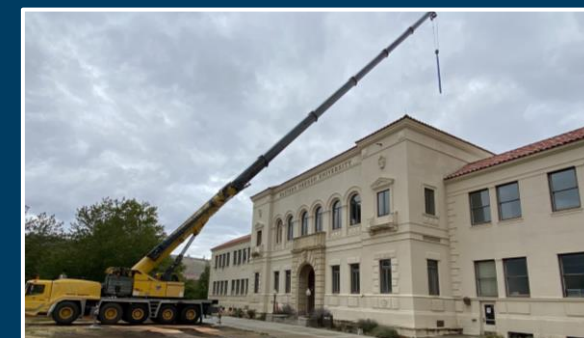
Eastern Oregon University Renovations
