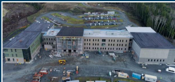
Seaside High School Construction Seaside, OR
