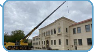
Eastern Oregon University Renovations, La Grande
