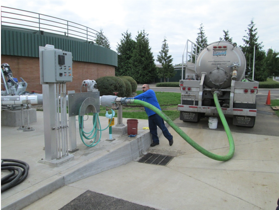
HOOKING UP HOSE TO UNLOAD A 5,000 GALLON LOAD OF FOG
