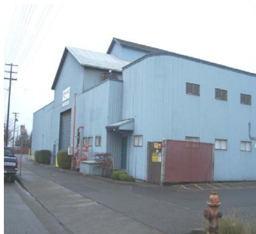
Painted Siding and Roof
