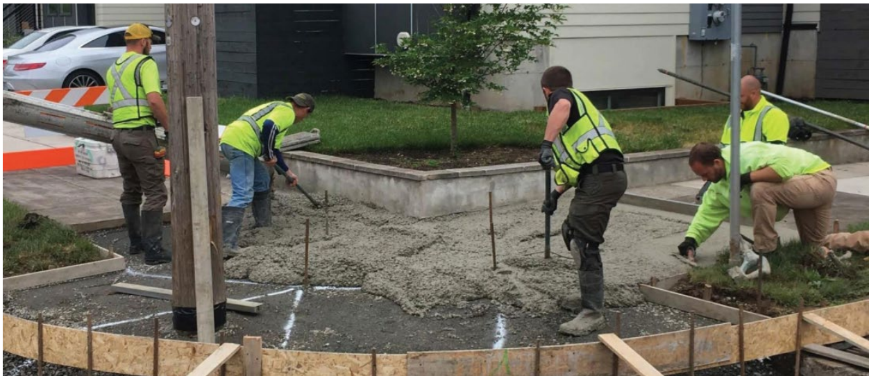
City of Portland's first round of low-carbon concrete pilot projects, featuring sidewalk ramps supported by DEQ.
