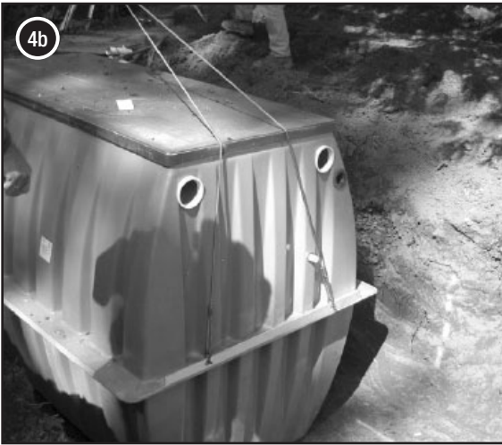
Lower the AX-RT unit into position.
