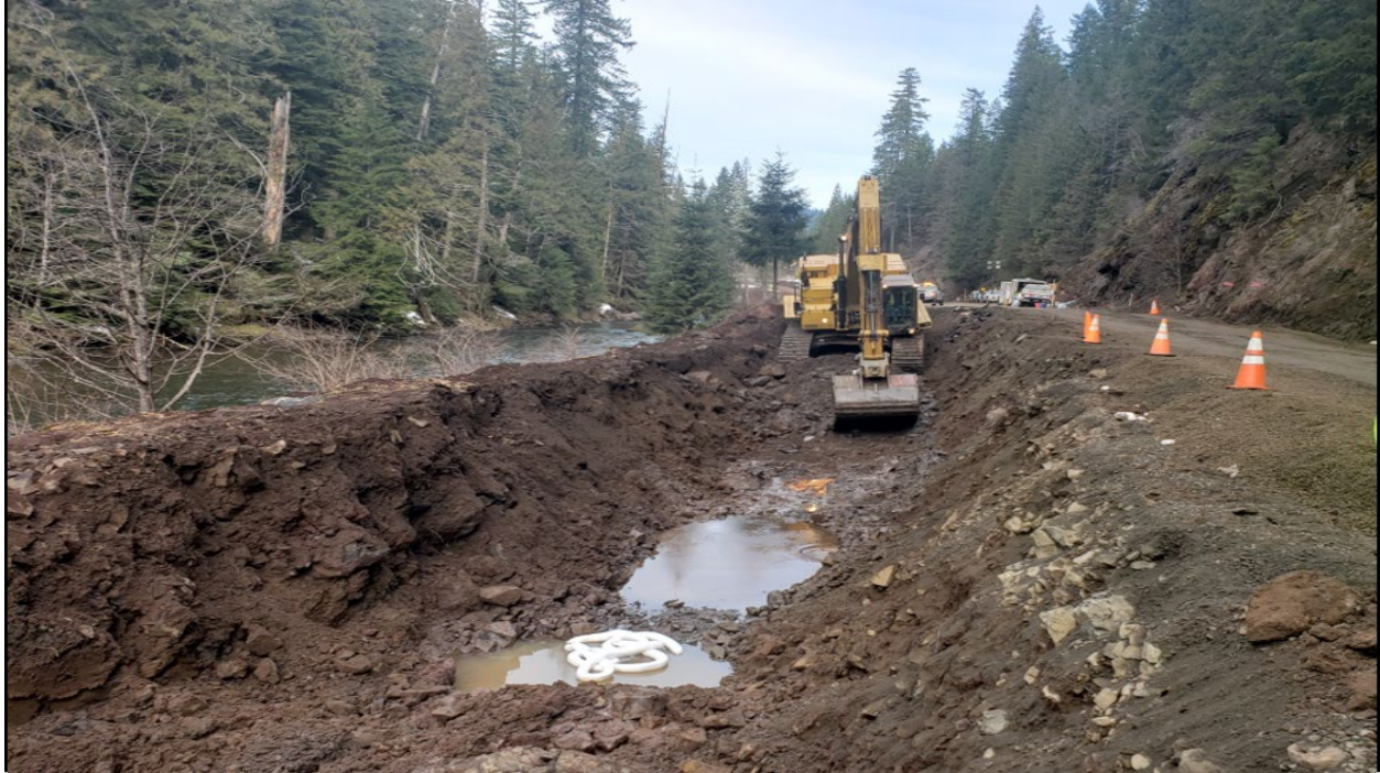
Figure 5 - Excavation to Groundwater Table - Bank Left Intact
