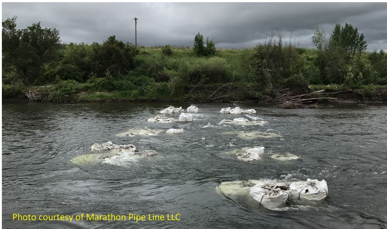
Figure 7 - Bags of Grout Stabilizing the Pipelines
