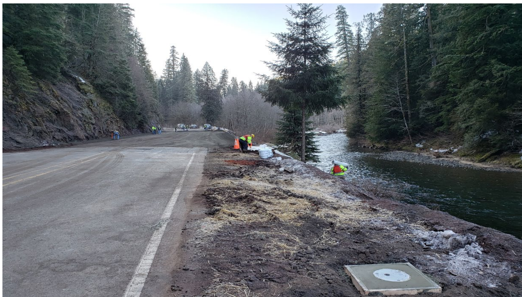
Figure 6 - Start of Highway Replacement
