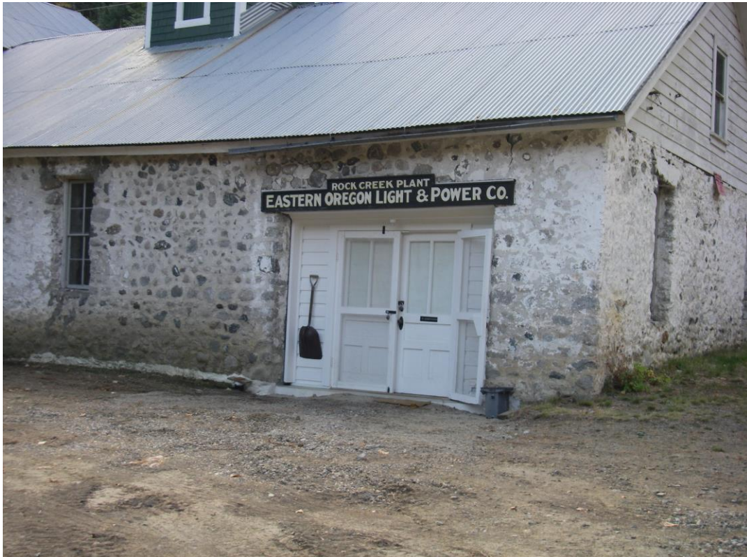
Figure 4. Historic Rock Creek Powerhouse.
