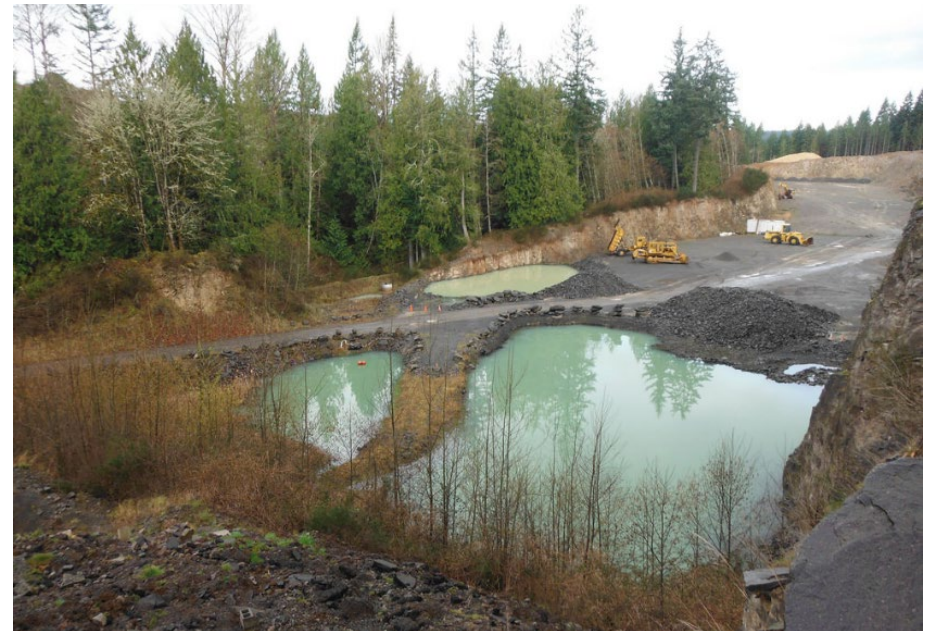
Stormwater control system at Graves Quarry in Molalla
