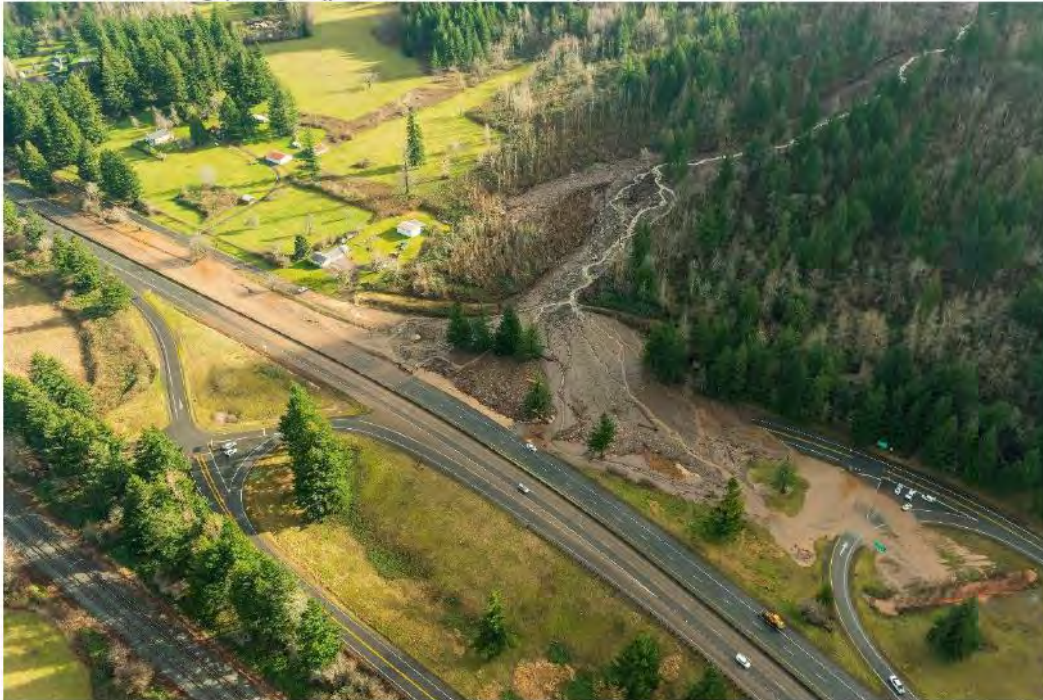
January 2021 Fatal Post-Fire Debris Flow. Source of debris flow within the 2017 Eagle Creek Fire, Columbia River Gorge, Oregon (photo courtesy of ODOT)
