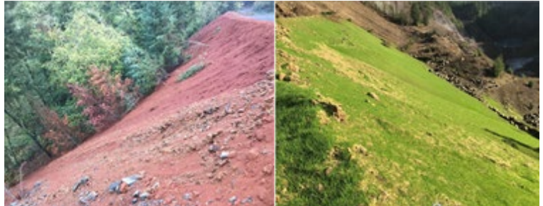
Slope before seeding
