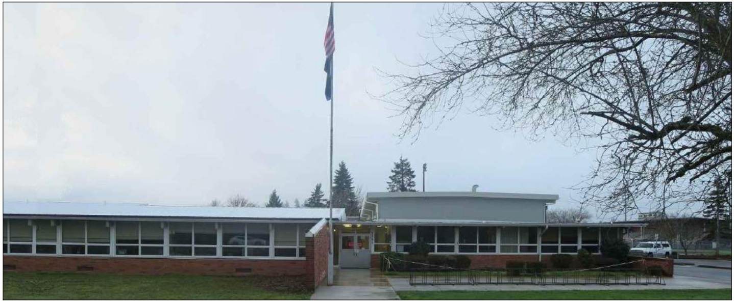
3 STREET ENTRANCE VIEW S0.0 NTS
