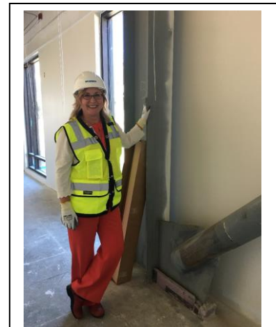
Figure 1. Dr. Lesley Ogden, hospital CEO standing next to robust steel members for the new resilient coastal hospital that opened in February 2020.
