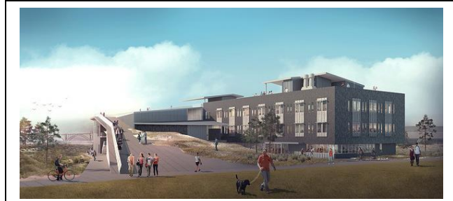
Figure 1. Image showing the wide ramp designed for tsunami vertical evacuation by many people to access the rooftop, which is designed to be above the tsunami inundation levels (Source: https://today.oregonstate.edu/news/osu-marine-studies-building-be-national-model-tsunami-“vertical-evacuation” )
