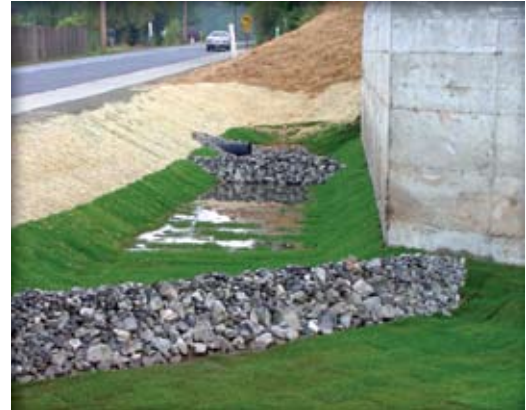
Developers are required to build on-site detention basins to handle increased runoff.
