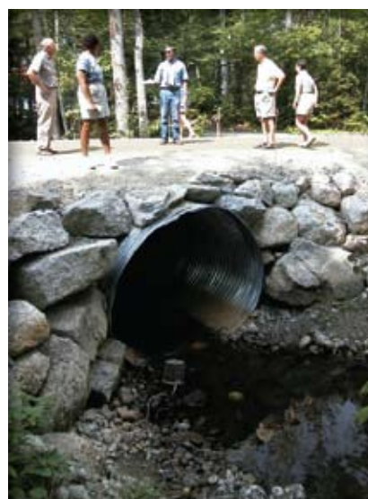
Culverts also require regular maintenance to keep floodwaters flowing freely
