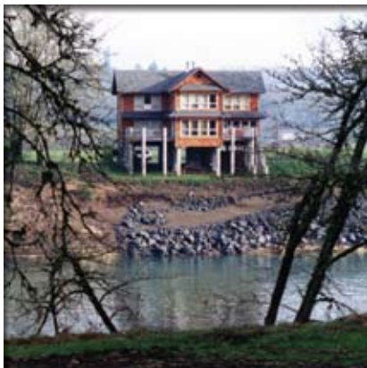
Elevated home in Douglas County, OR
