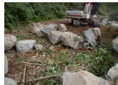
Adding rocks (boulders and gravel)
