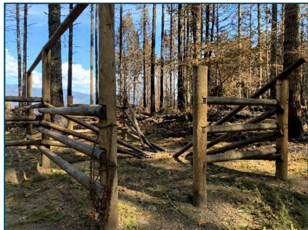
Photo 8. Horse Camp corral damage
