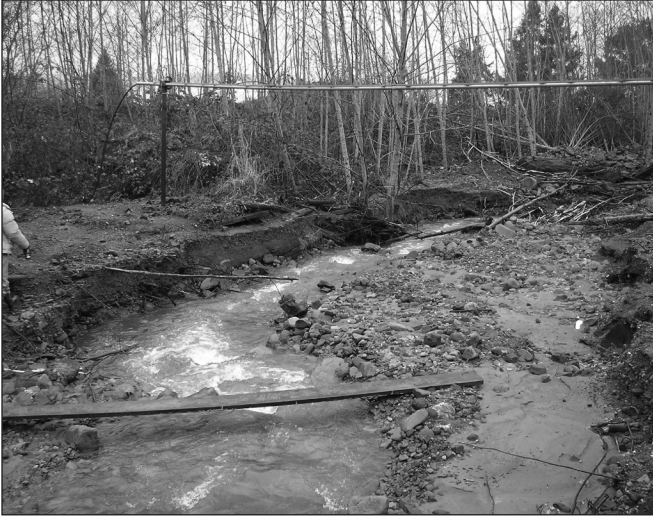
Washed out bridge and transmission line in Marshland.
