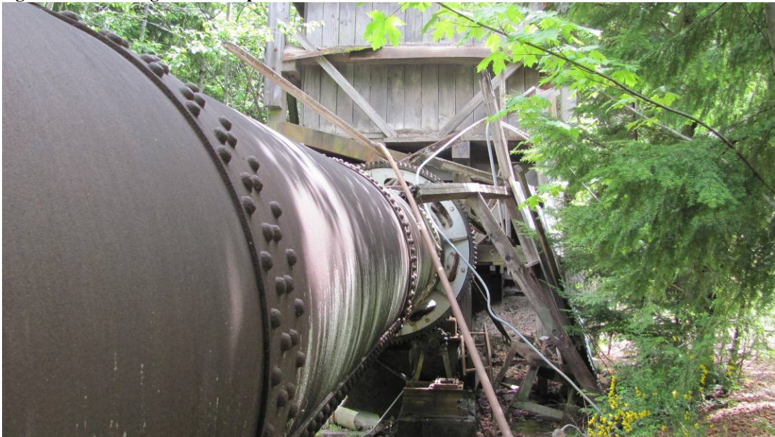
Figure 8. Remaining structural pieces of New Furnace
