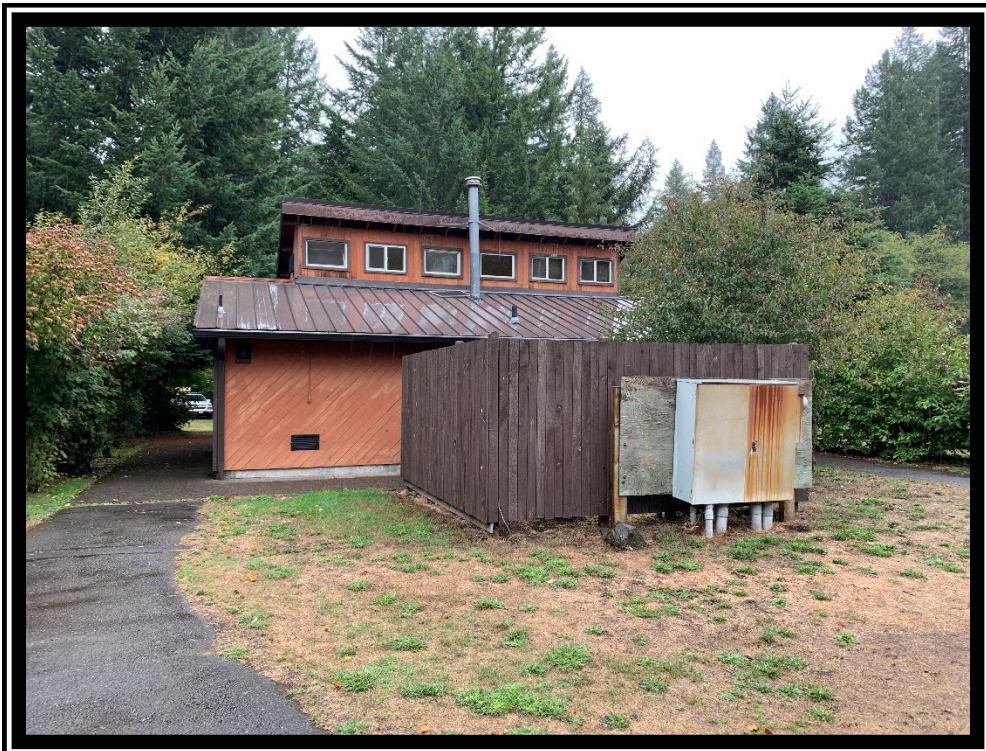
Figure 2 – Existing infrastructure corral adjacent to restroom.
