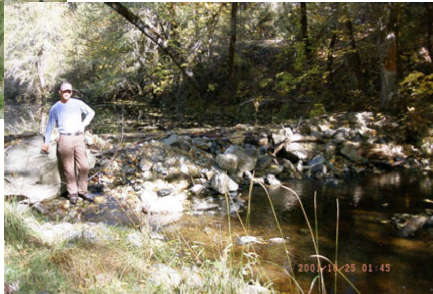
Evans Creek Push-Up Dam (2001) Push-Up Dam on Evans Creek Used for Recreational or Aesthetic Purposes No Fish Passage
