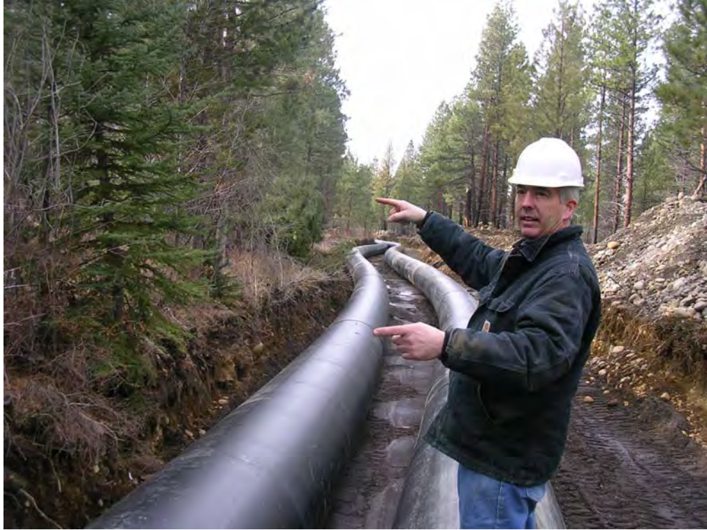
Three Sisters Irrigation District Piping 210-4023-7705
