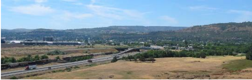
The Chenoweth Interchange on I-84 west of The Dalles, OR.
