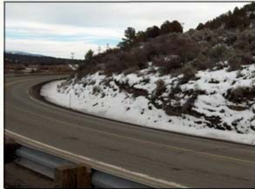
A sharp corner in the Beatty Curves area.
