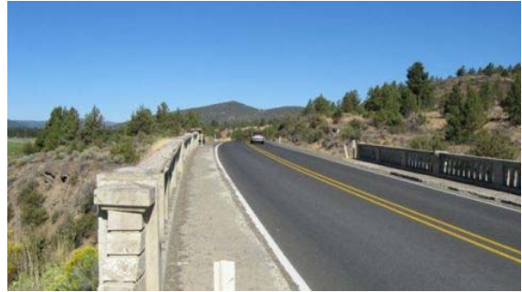
The Dairy Bridge on OR 140 looking east.
