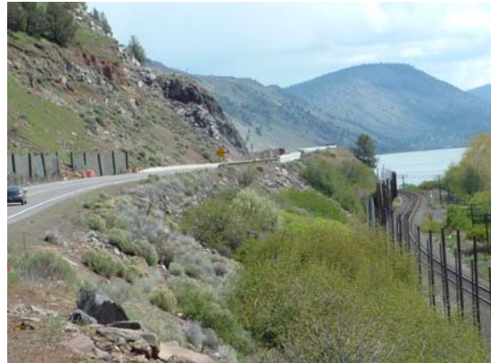
US 97 near Modoc Point looking south.
