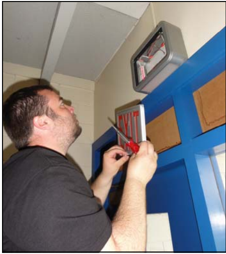
Neil Oliver, LCC student auditor, checks to see the type of light used in the exit sign at Malabon Elementary in Eugene. The audit is part of the Governor's School Energy Audit Initiative paid for with Recovery Act funds.
