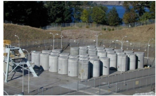
34 casks store spent fuel at the former Trojan Nuclear Power Plant site.
