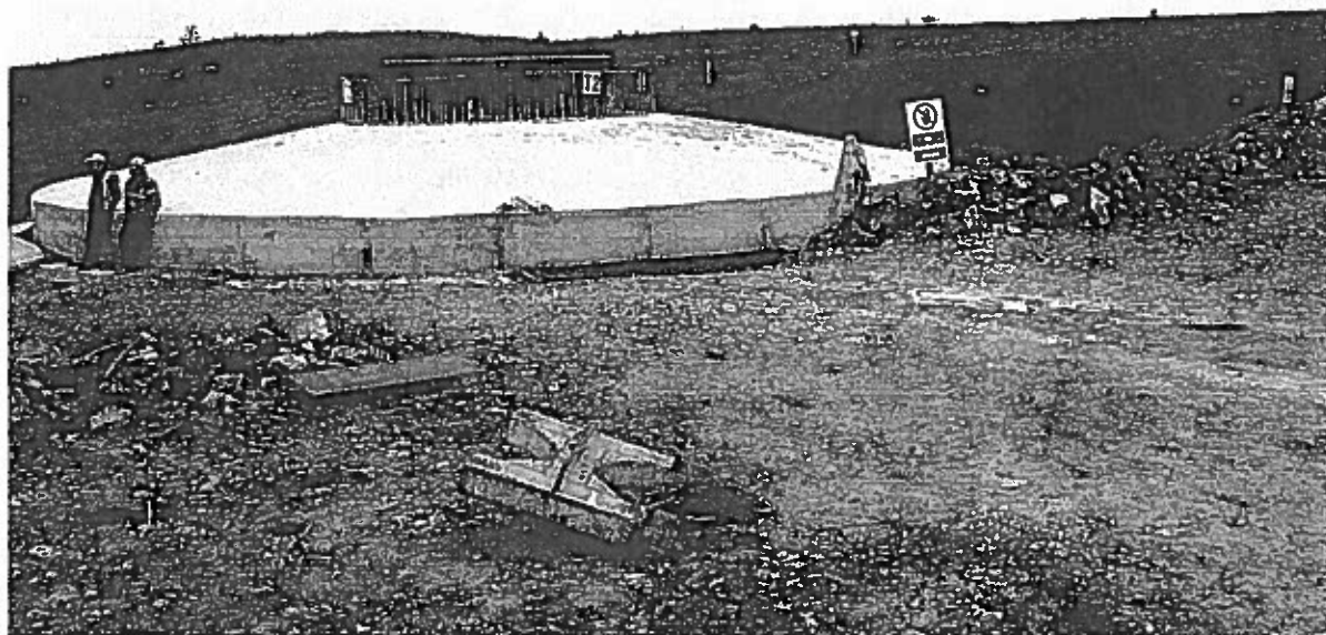
Figure 1: Construction of the foundation of a single wind turbine.
