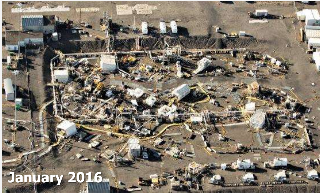
C Farm before & after completion of waste retrieval
