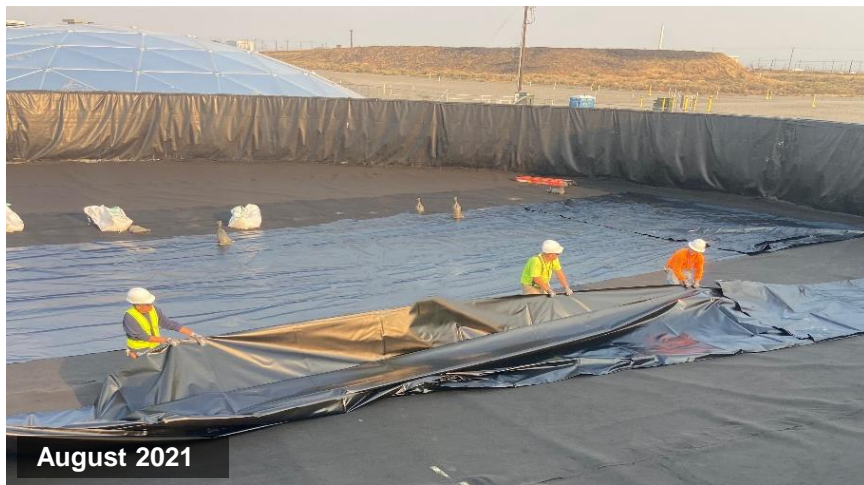
Integrated Disposal Facility leachate tank liner installation
