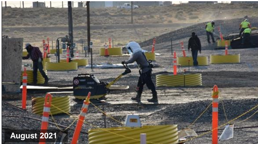
TX Tank Farm interim surface barrier installation
