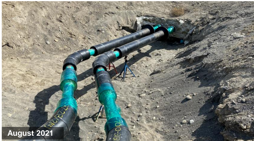
Newly installed waste feed delivery lines between AP Tank Farm and the Low-Activity Waste Facility
