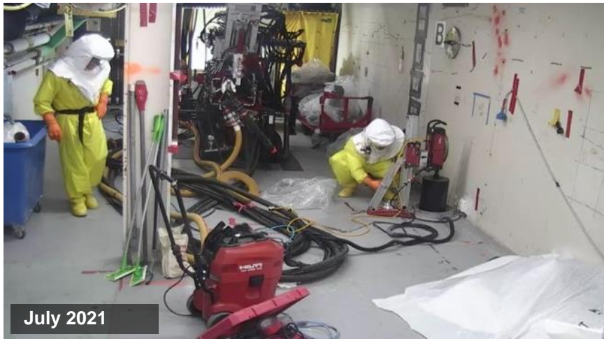
324 Building micropile preparation
