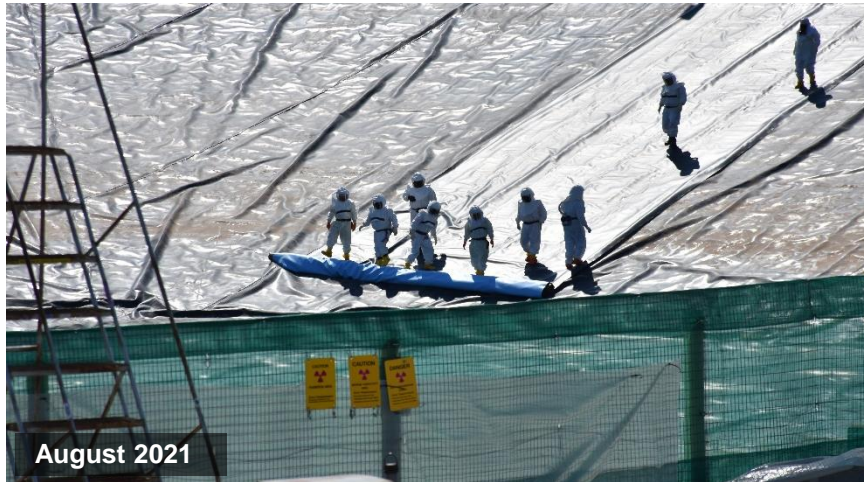
Installing replacement cover on Basin 44 of the Liquid Effluent Retention Facility
